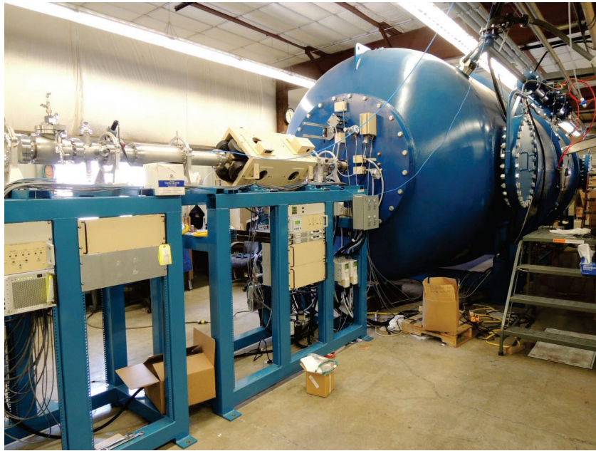
Figure 1. Photograph of setup for the high-voltage test at NEC, USA in January, 2014.
